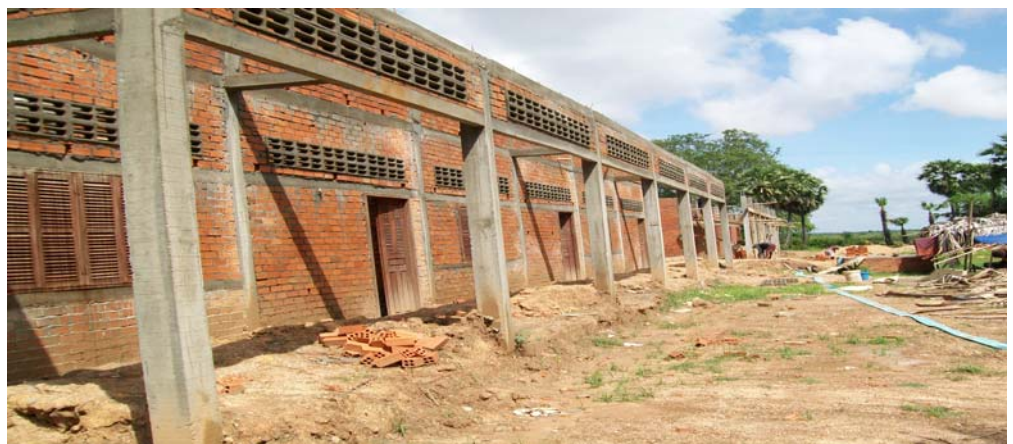
New Schools 2010 under construction.
